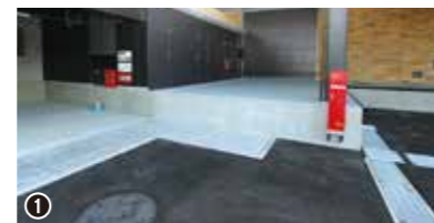
1 Loading bay for Medium Hall
