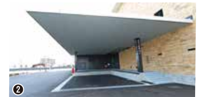
② Loading bay for Grand Hall
