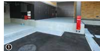
① Loading bay for Medium Hall
