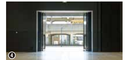
④ Loading entrance for Exhibit Hall (view from inside)
